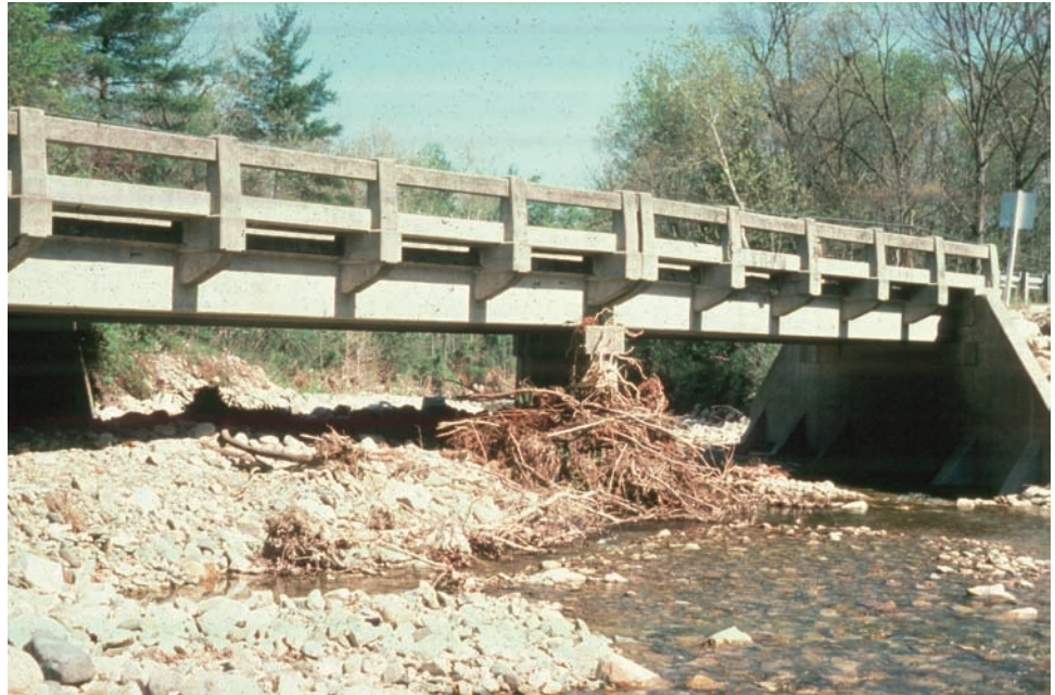
Figure P.2.27 Integral Bridge
