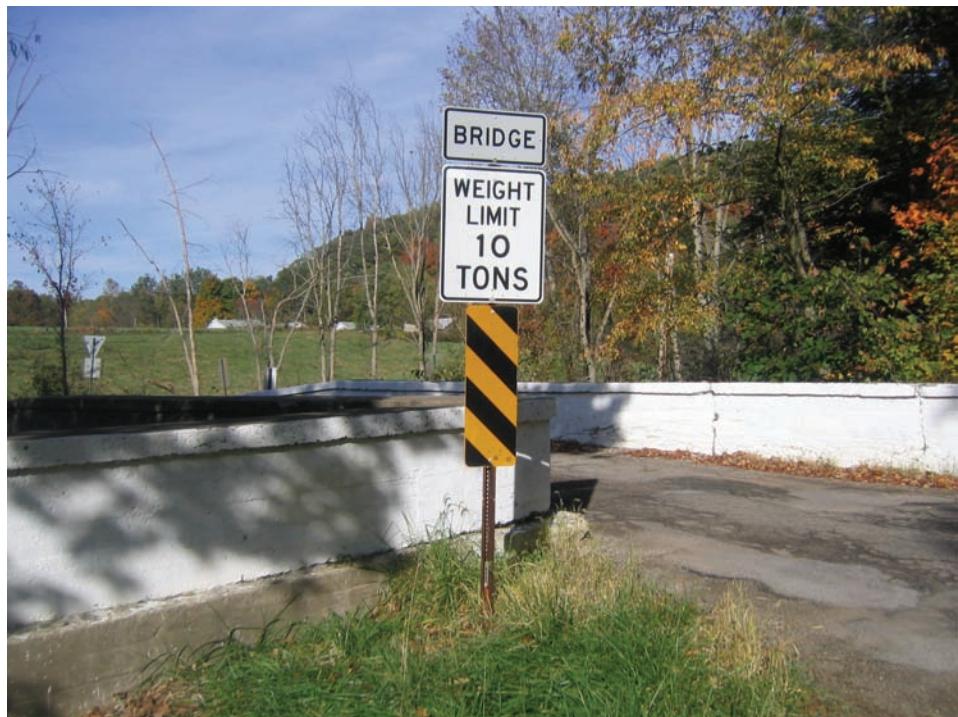
Figure P.2.20 Bridge Weight Limit Posting
